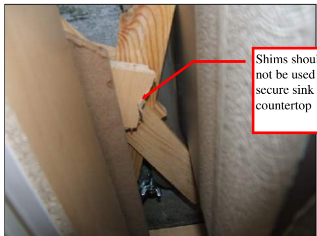
Improperly secured kitchen sink
