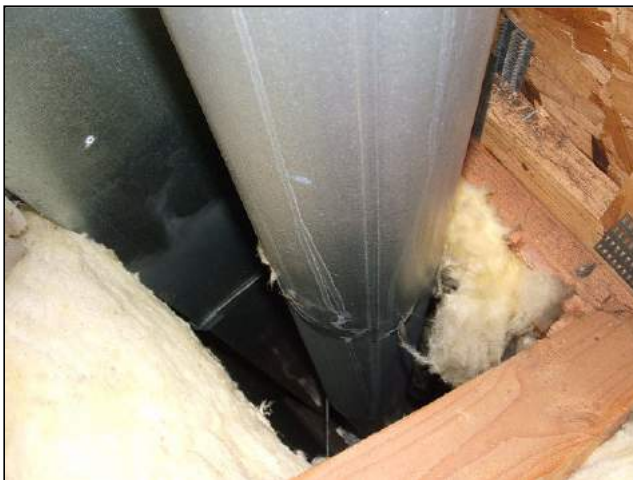
Improper fire stop around chimney
