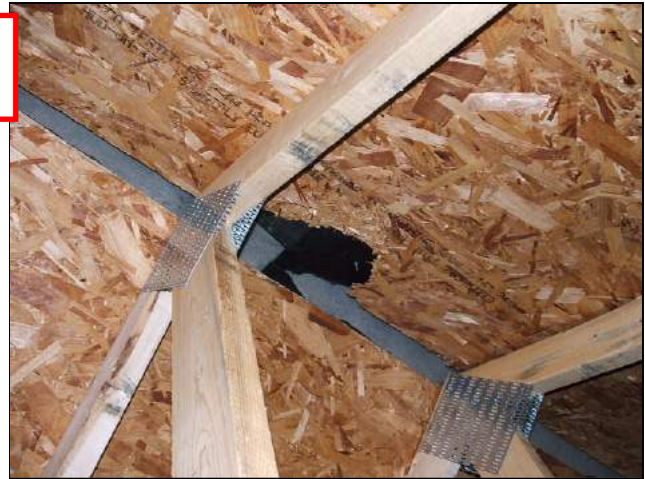
Damaged sheathing
