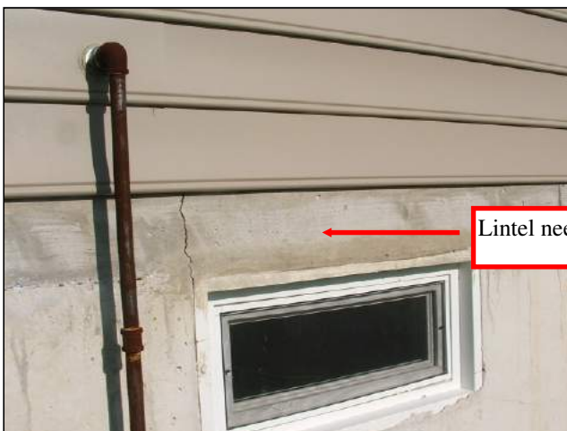
Crack due to improper window support
