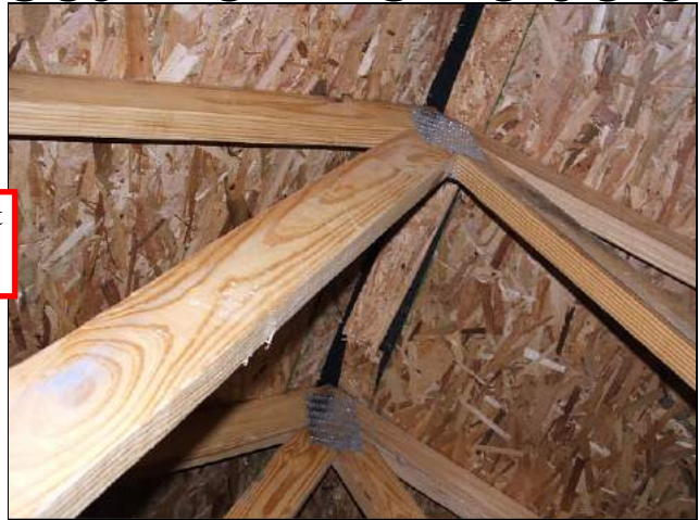
Damaged sheathing
