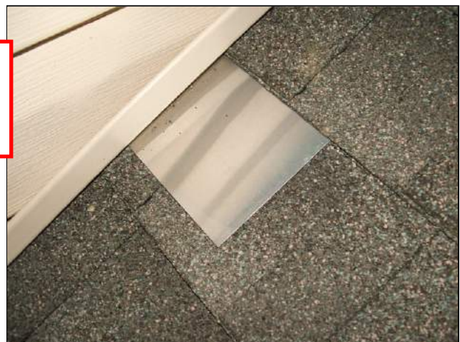
Improper flashing at roof/wall intersection
